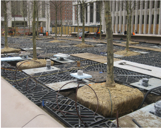
Custom metal decks were used around the tree openings to make the lights work in the thinner paving.
